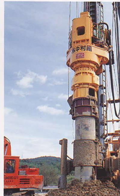
SMD-200H Pier expansion work steel pipe pile
