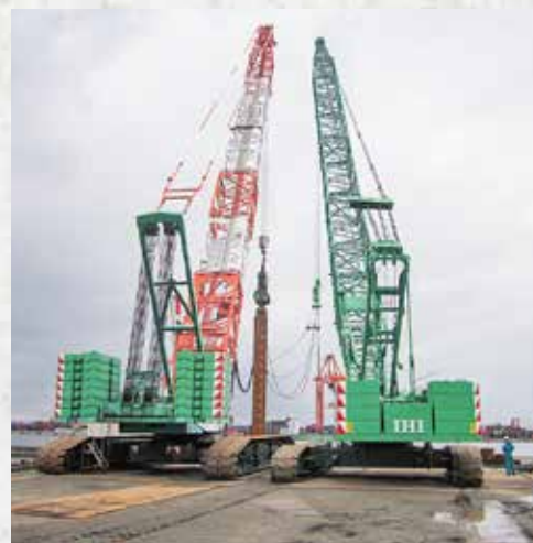
Impact hammer combined with waterjet driving method
