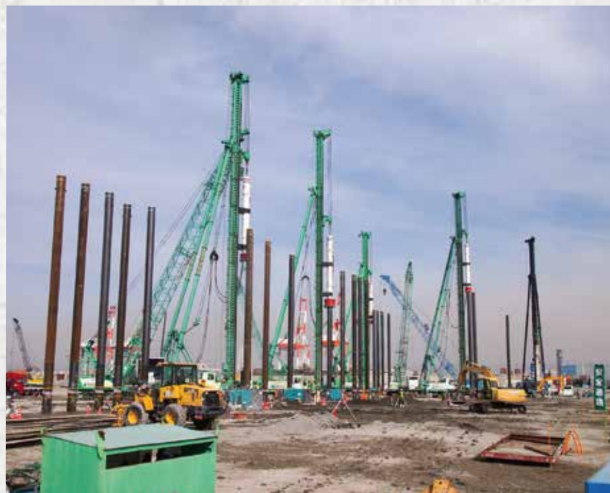
Impact hammer driving method
