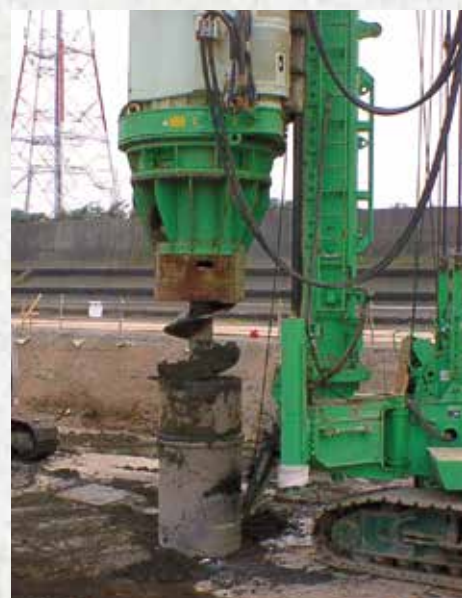
Doughnut auger method
