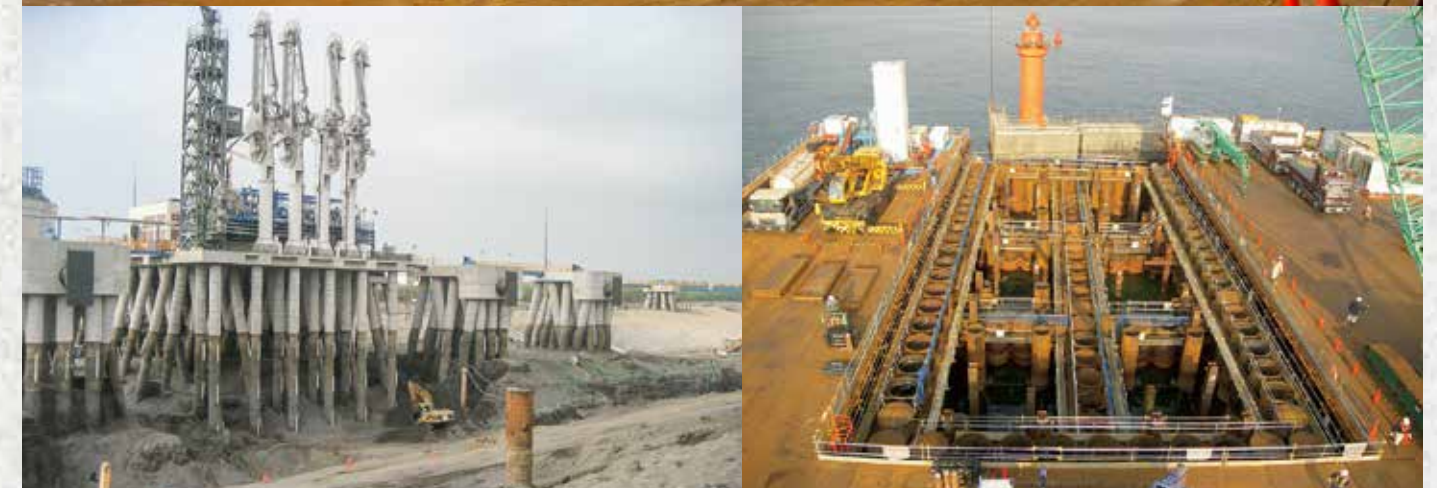
Driving with vibratory hammer and finish striking with impact hammer method
