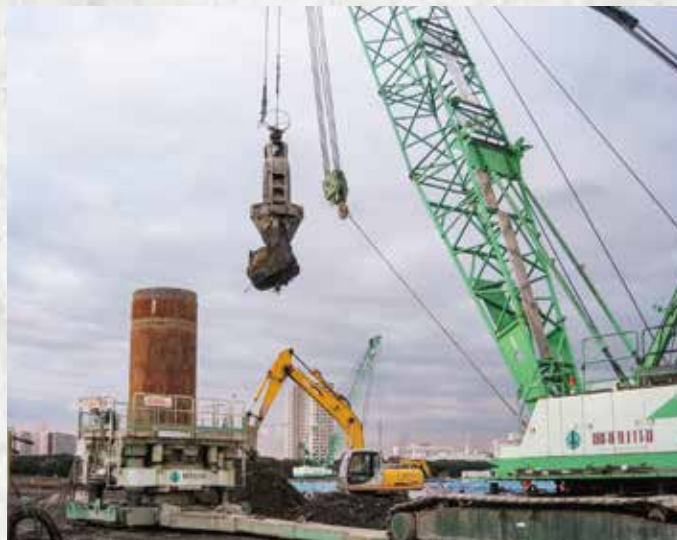
Super top method (Obstruction removing)
